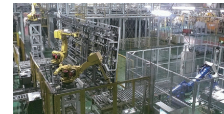
Coating (on an unmanned coating line)
